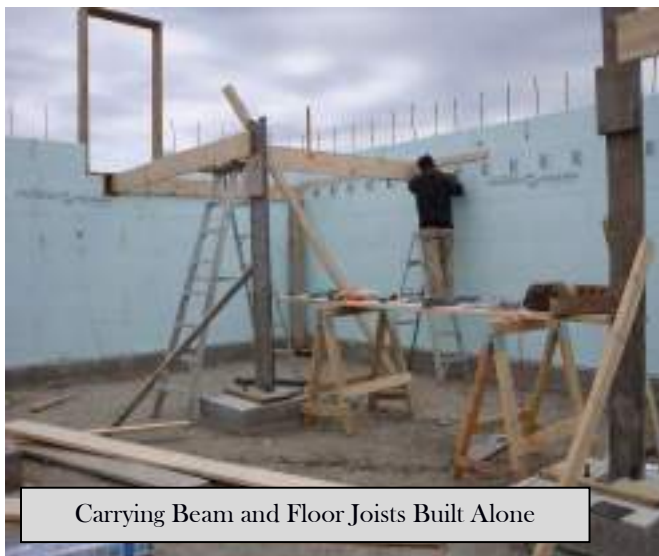
Building Main Carrying Beam and Floor Joists Nova Scotia
